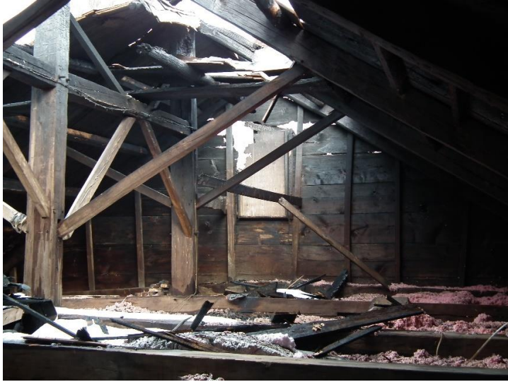
Attic, looking east.
