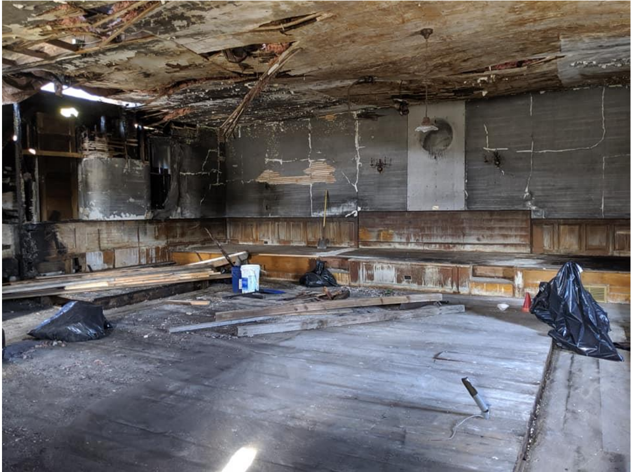
Interior of second floor looking east toward the altar platform.
