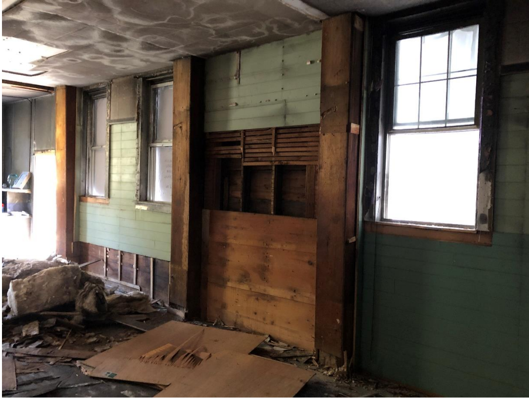
Interior of first floor during (above) and after (below) selective demolition, looking south where former central entrance was. The green beadboard was applied atop the original plaster and wainscot.
