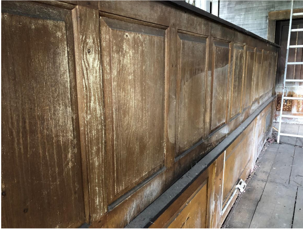
Paneling in the sanctuary, recycled from the 18 th c. gallery breast work.
