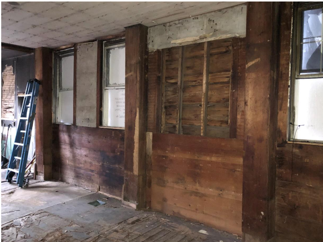
Interior of first floor during (above) and after (below) selective demolition, looking south where former central entrance was. The green beadboard was applied atop the original plaster and wainscot.
