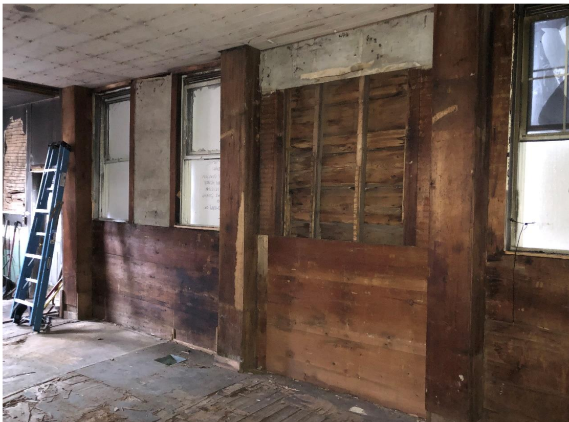
The interior of the Grafton Center Meetinghouse shows that the wood was left unpainted.
