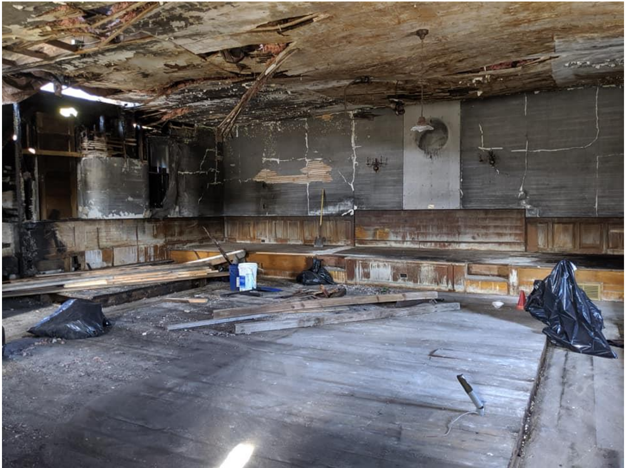
First floor space, looking NE toward altar platform.
