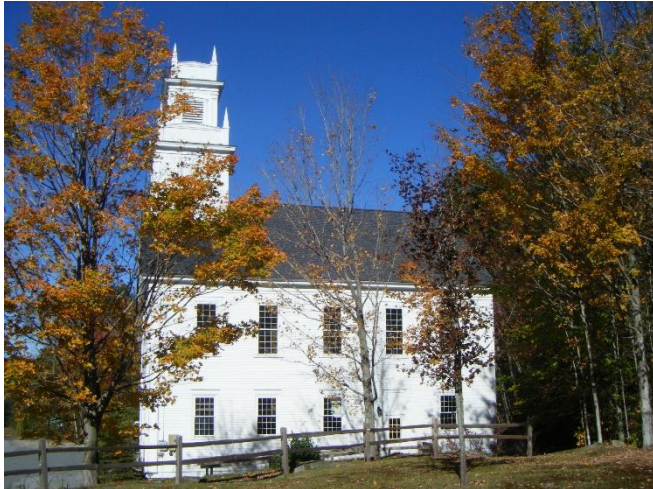
Springfield Meetinghouse, built 1797, renovated 1851.
